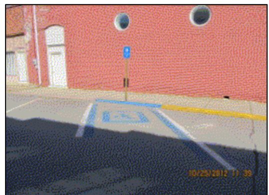
Photo illustrates on-street angled parking on W. 3 rd St. No access aisle is painted and sign is too low.
