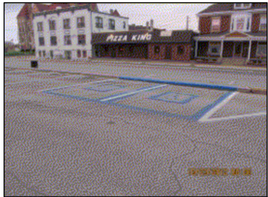
Public parking lot spaces with no access aisles or signage.
