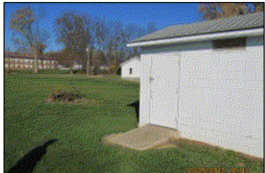
Community Park restrooms are not on an accessible route and have no level landing at the entrance door.
