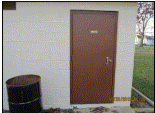
South Memorial Park restroom with non-compliant sign and step into door.
