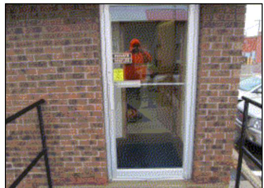
City Hall side entrance has glass within 10" of the bottom of the door.
