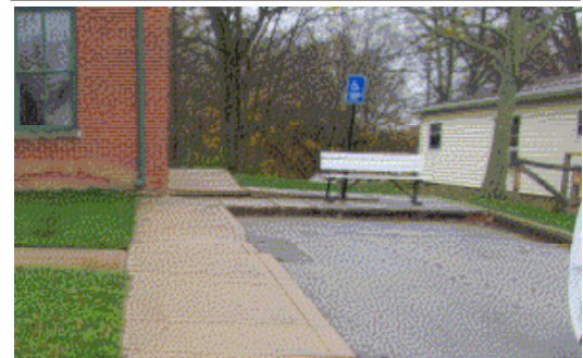
Non-compliant parking space and bench in sidewalk to ramp at the Community Center.
