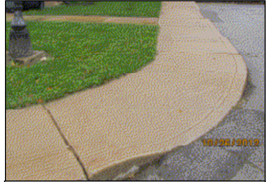
Non-compliant ramp creates cross slope issues along walk.
