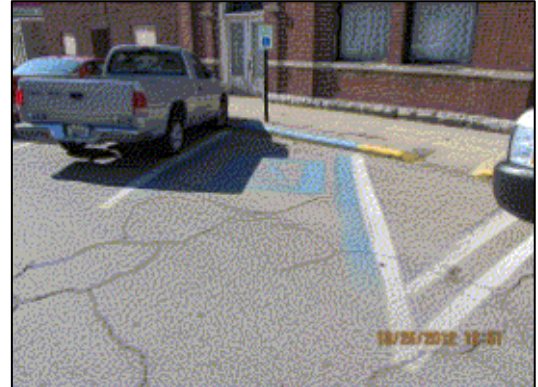
Photo illustrates on-street angled parking on N. Morgan St. Access aisle is not marked and space available is not compliant. Also note the curb ramp is not 48" width.
