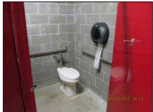
Riverside Park women's stall is too narrow, toilet paper dispenser is over the short side grab bar, and flush control is not on the wide side of the toilet
