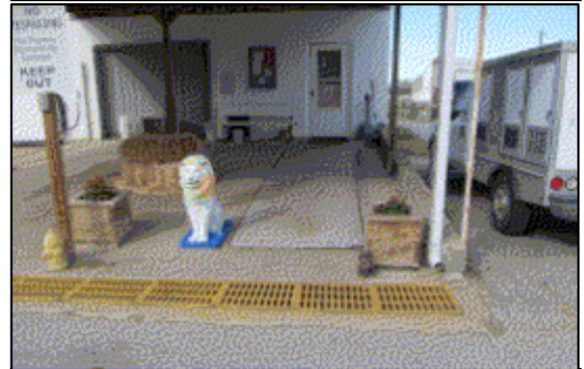
Animal Shelter approach walkway includes trench drain with large openings.
