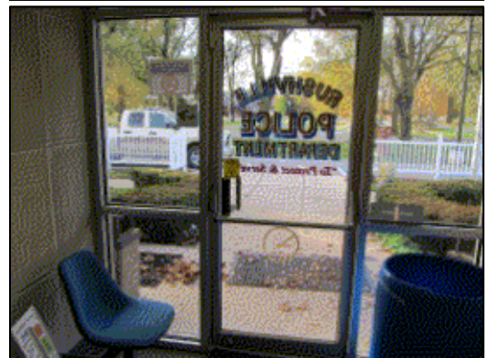
Police Department entrance has glass within 10" of the bottom of the door.
