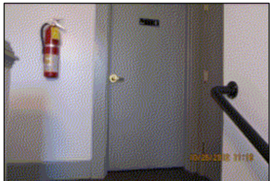
Protruding fire extinguisher.
