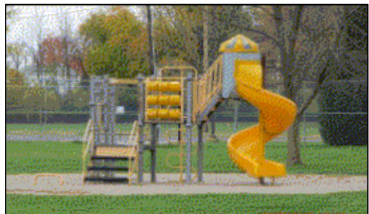
Community Park play structure is not on an accessible route, transfer platform does not comply, and surfacing is not accessible.
