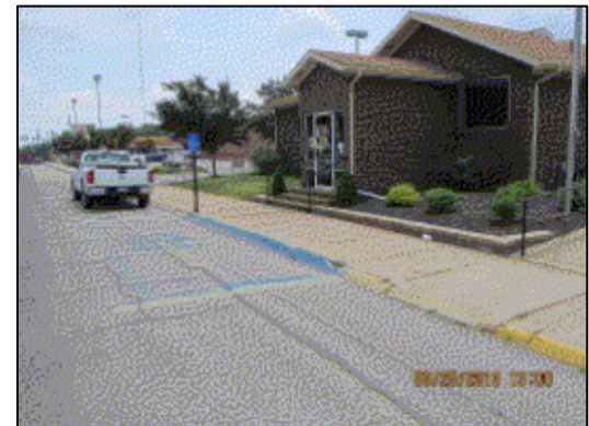
Photo illustrates on-street parallel parking at City Hall. Sign is too low.
