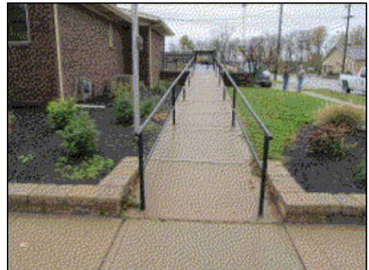
Non-compliant exterior ramp at City Hall.
