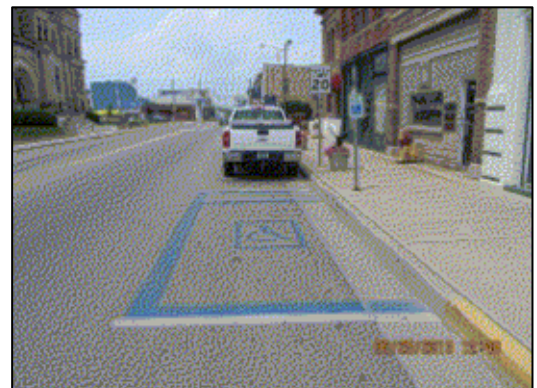
Photo illustrates on-street parallel parking on E. 2nd St. Sign height is too low.
