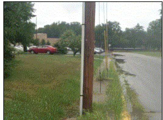
Example of obstruction narrowing sidewalk width to under 48" minimum required.
