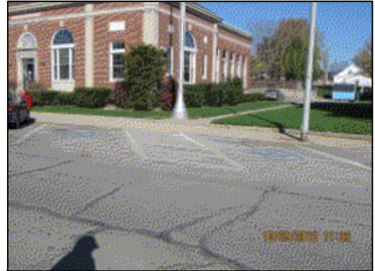
Photo of angled parking at the Post Office. Access aisle is not wide enough and there are no signs present.
